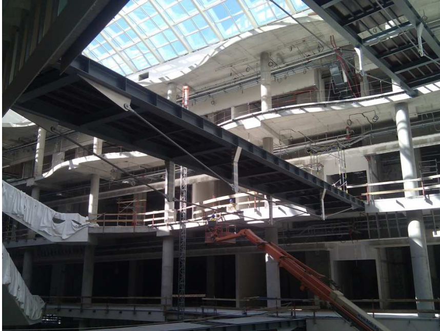
The finishing works are underway
