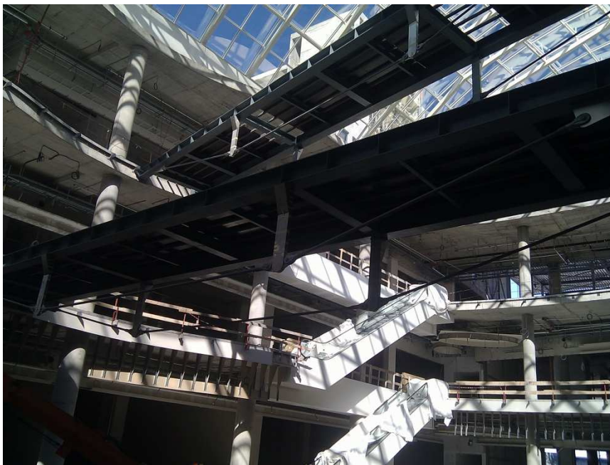
The footbridges seen from ground zero
